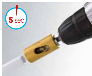
2- Chamfering the pipe
