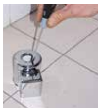
4. Create the correct space to connect the trap
