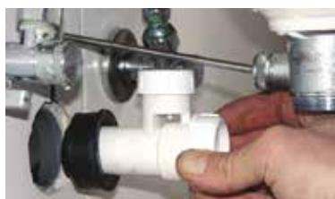
2. Install the AAV with technical gasket
