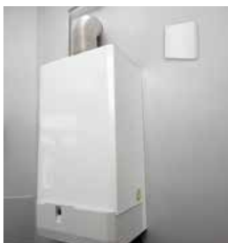
Bathrooms & rooms with boilers
